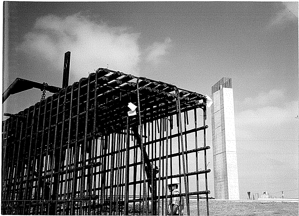
Figure1.2 Cage of Bent Cap
