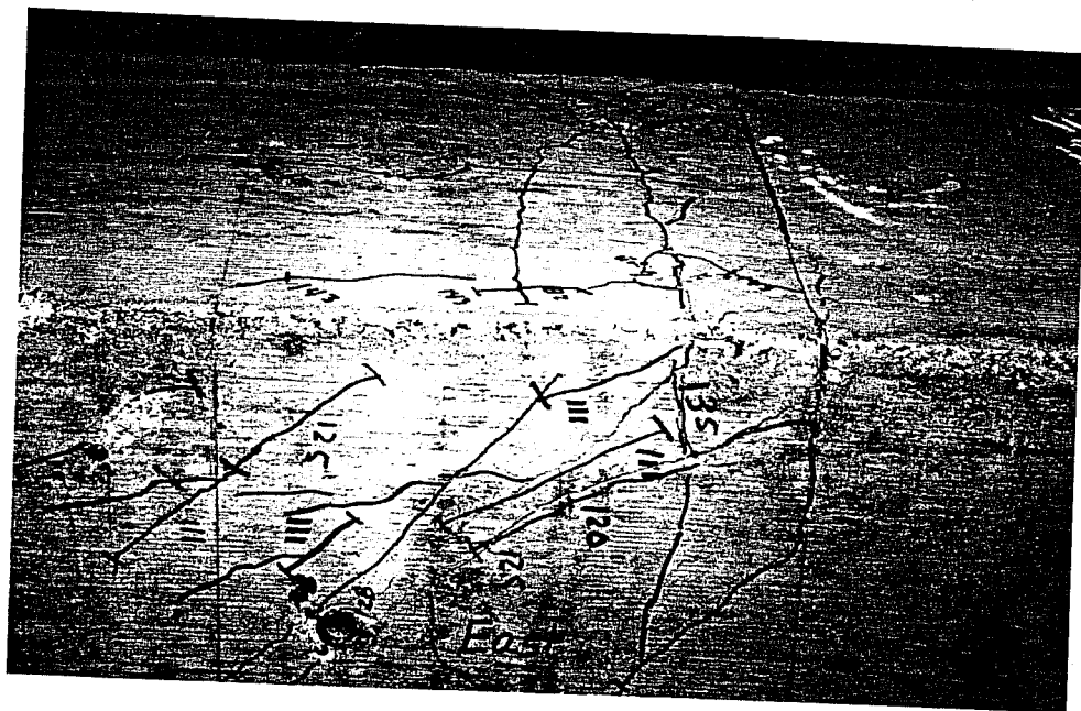
Figure 4.20 Failure mode of two layers of bundled bars with transverse reinforcement, --Shear in anchorage zone (Test 16 2-16-S-B)
