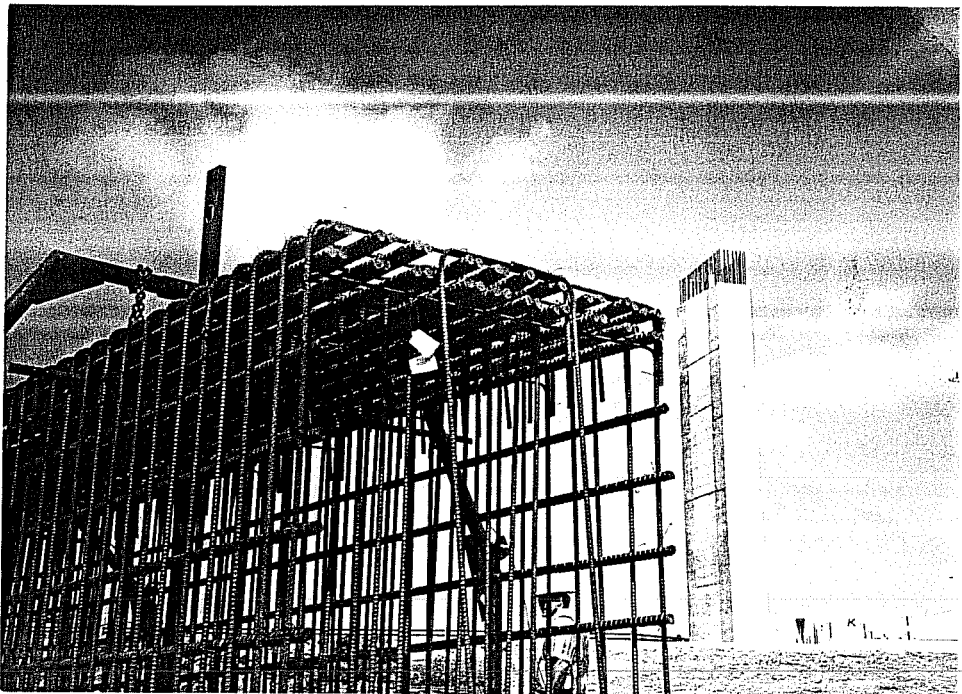
Figure1.2 Cage of Bent Cap
